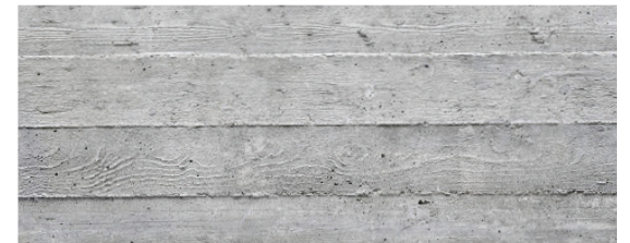
Board Formed Concrete
