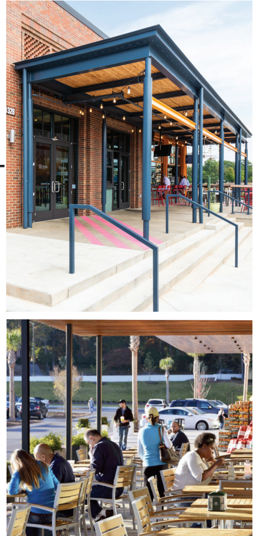
Side Porches and Canopies
