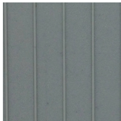
Standing Seam Roof
